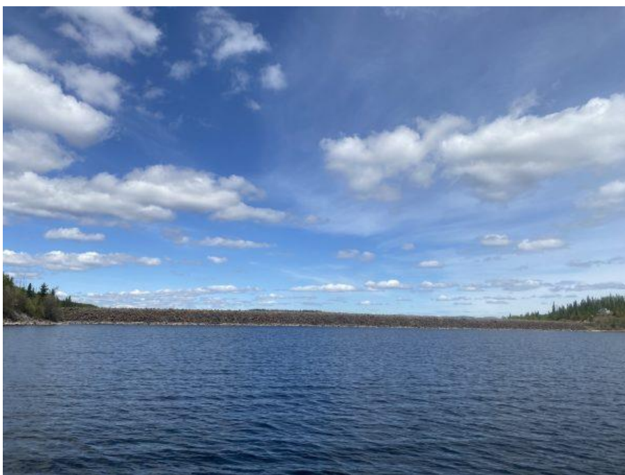
Kenney Dam south of Vanderhoof from the water
